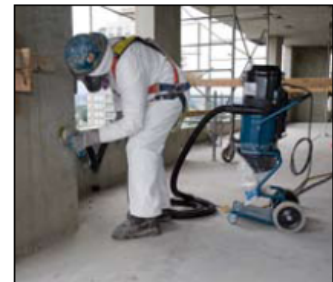
Worker grinding concrete using local exhaust ventilation
