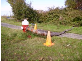
1. Ex. Water Main Flushing
