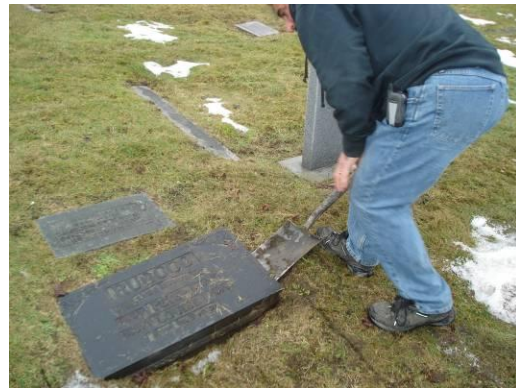
Removing marker prior to repair
