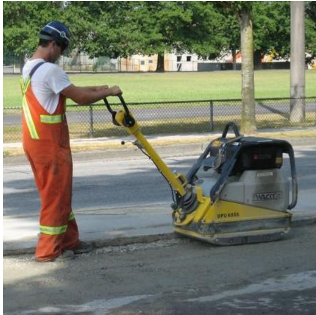
Figure 8: Ops III worker tamping the site after work completed.
