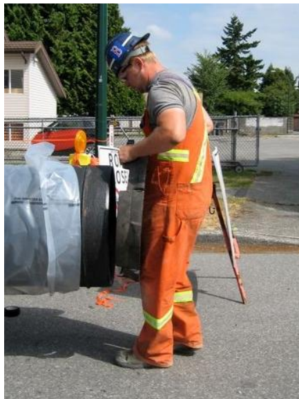
Figure 5: Ops III worker attaching a fitting to large diameter pipe.
