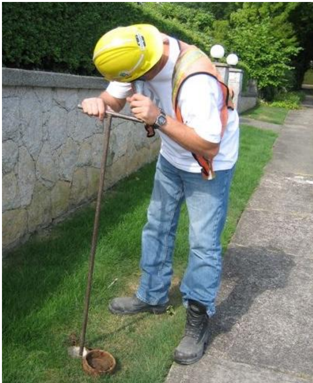
Figure 1: Ops III worker listening for a leak through the leak phone placed against service key.
