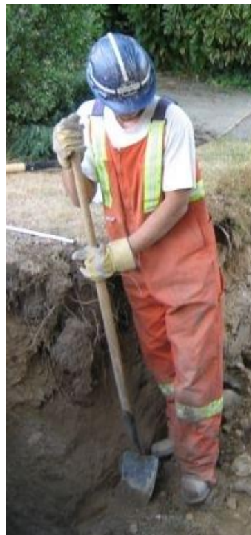
Figure 2: Ops III worker hand digging.
