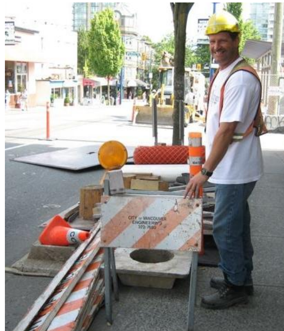
Figure 7: Worker with barricades to divert traffic.
