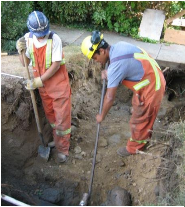
Figure 6: Ops III worker and sub-foreman hand exposing lines.
