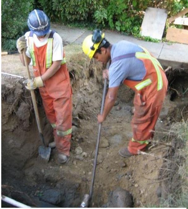
Figure 7: Ops III worker and sub-foreman hand exposing lines.
