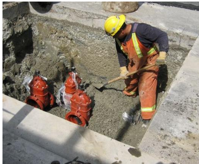
Figure 10: Ops III worker shovelling cement to create thrust block.
