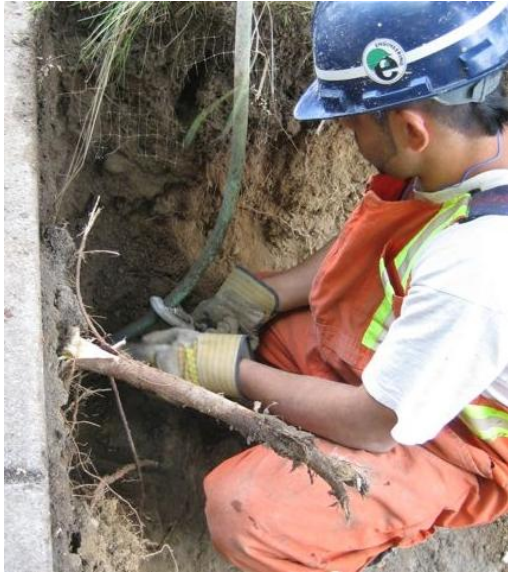
Figure 3: Ops III worker cutting ¾” copper service pipe with a pipe cutting tool.
