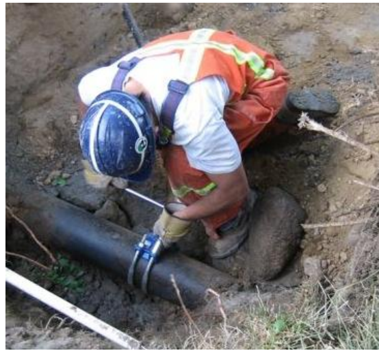
Figure 2: Ops III worker attaching service saddle to main.
