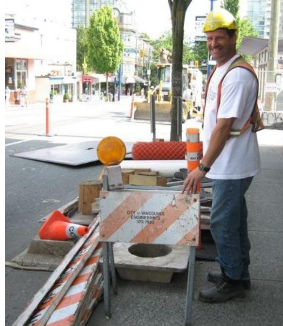
Figure 8: Worker with barricades to divert traffic.
