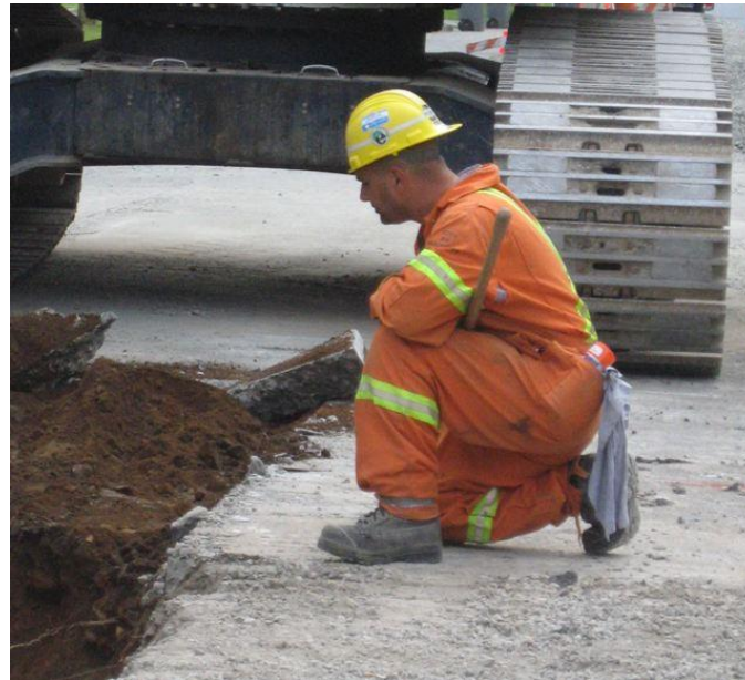
Fig. 15: Padman monitoring pipe laying in ditch.
