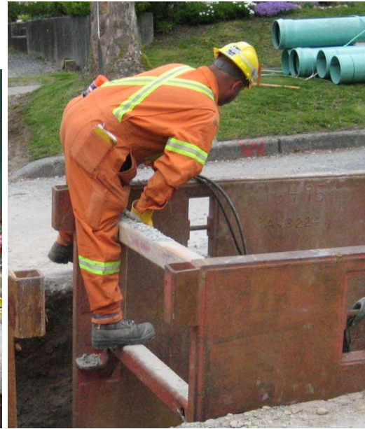
Fig. 9: Attaching cables to cage for moving it.
