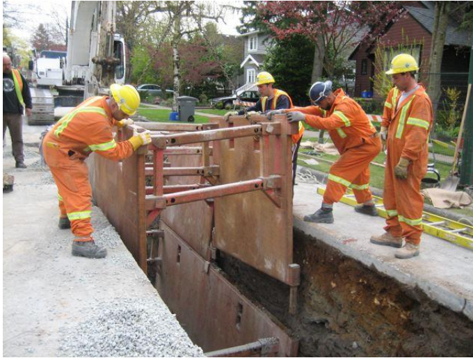
Fig. 8: Guiding steel cage into place.
