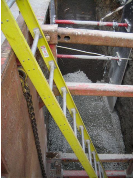
Fig 10: Typical ladder positioning in ditch
