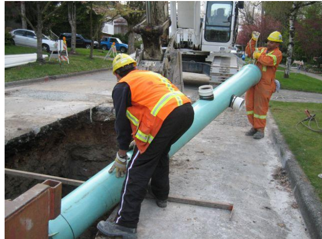
Fig 4: Lowering pipe into ditch with rope chain.
