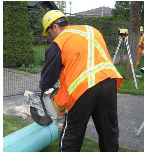
Fig 2: Cutting PVC with chop saw.
