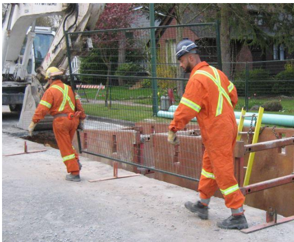
Fig. 12: Carrying fences to safeguard ditch.
