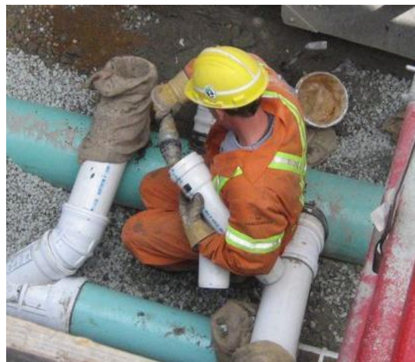
Fig 6: Lubricating bend before connecting it.
