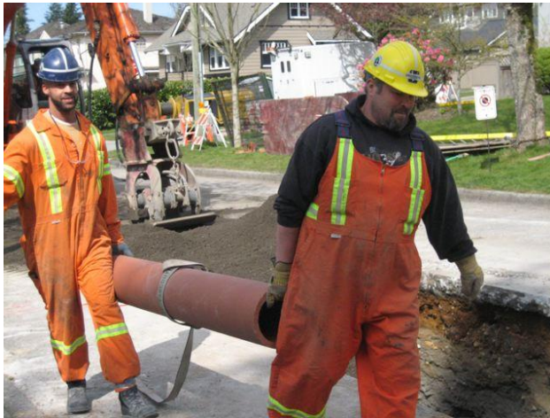
Fig 1: Carrying VIT pipe
