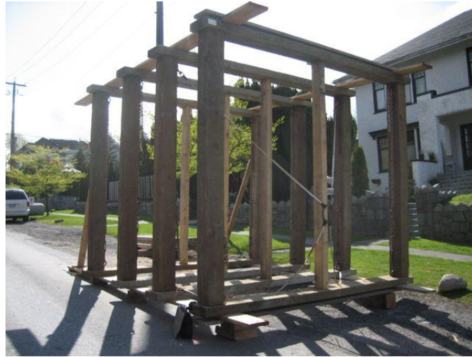
Fig 11: Timber set fully constructed.
