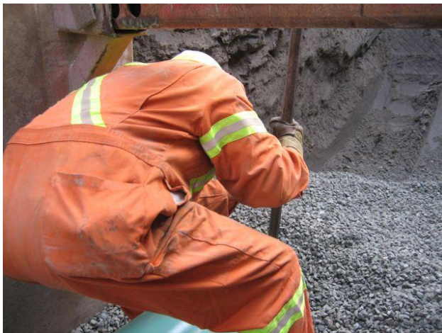
Fig 5: Levering pipe into place with probe bar.
