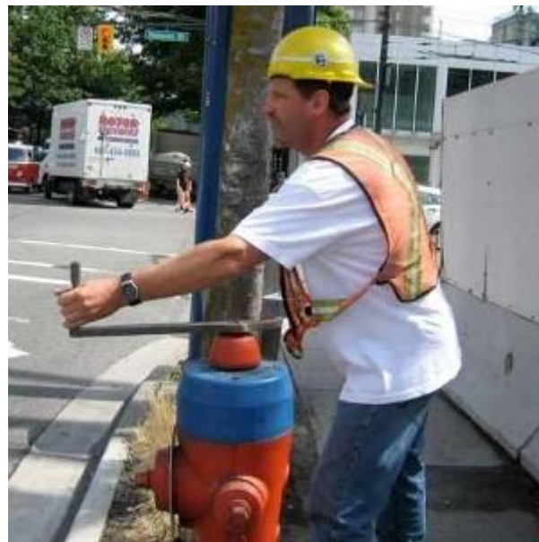
Fig. 8: File photo of a city worker opening a hydrant using a hydrant wrench.
