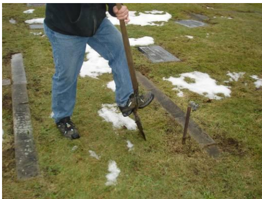
Digging hole around stand pipe
