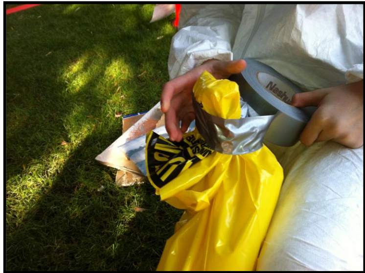
Instating a Goose Neck Seal on the Waste Bags
