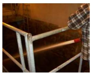
Photograph 1. Worker washing the walls of the wet well – 225<sup>th</sup> Street Sewer Lift Station.
