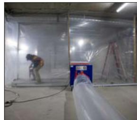
Worker drilling concrete inside an enclosure equipped with a "negative air" unit
