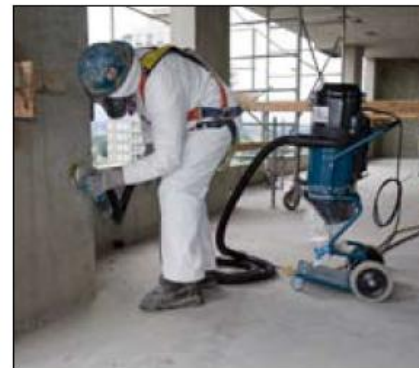
Worker grinding concrete using local exhaust ventilation
