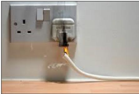
Power cords become frayed or damaged from heavy use and age and should be inspected regularly.
