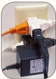
Overloaded electrical outlet
