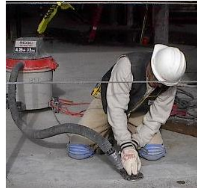
Concrete sander with local HEPA exhaust ventilation
