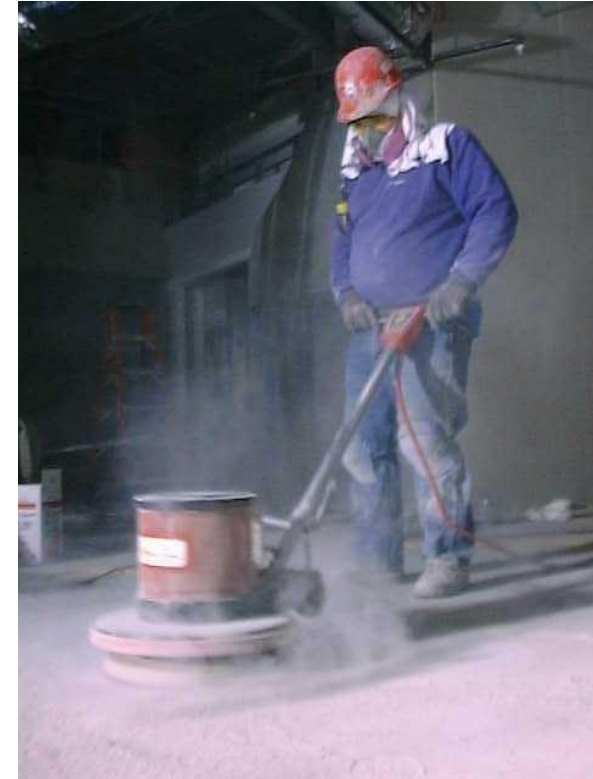
Concrete sanding / grinding
