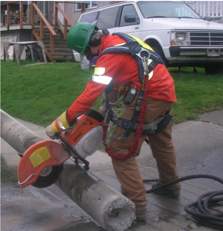
Wet cutting of concrete pole
