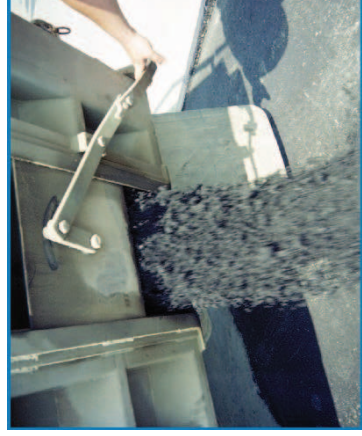
Push down on pull-up door to release asphalt
