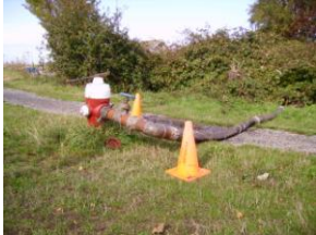
1. Ex. Water Main Flushing
