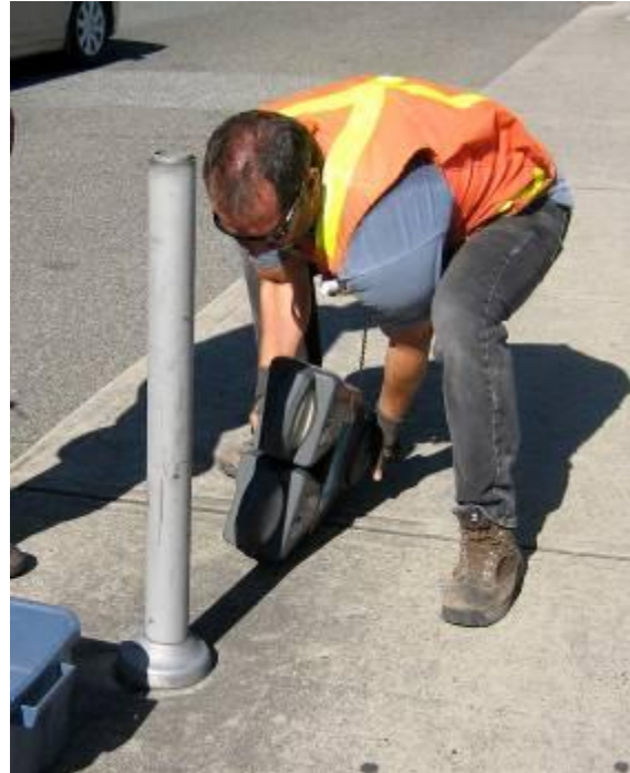
Fig. 13: Removing meter head to tighten post.
