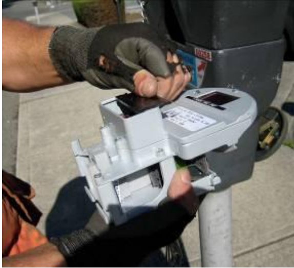
Fig. 3: Replacing meter batteries.
