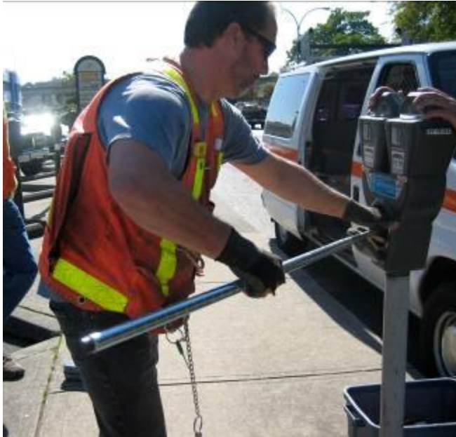
Fig. 12: Using wrench to loosen main bolt prior to removing meter head.
