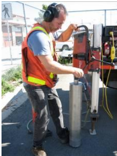
Fig. 21: Coring drill in use.
