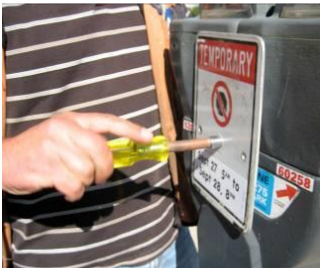
Fig. 8: Installing meter hoods, decal applied on bottom of hood.
