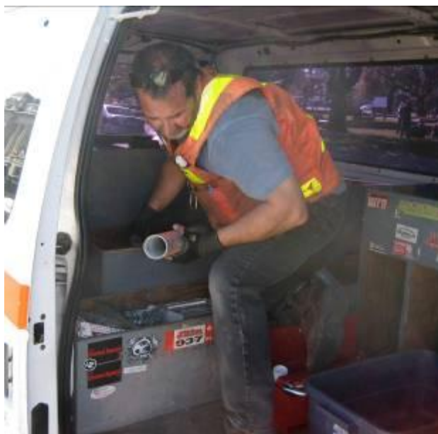
Fig. 22: Carrying a post out of the van for installation.
