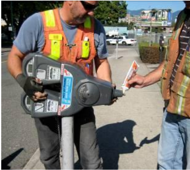
Fig. 23: Greasing the head before installation.
