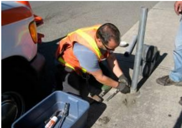
Fig. 14: Inserting wedges and replacing bolts to tighten a meter post.
