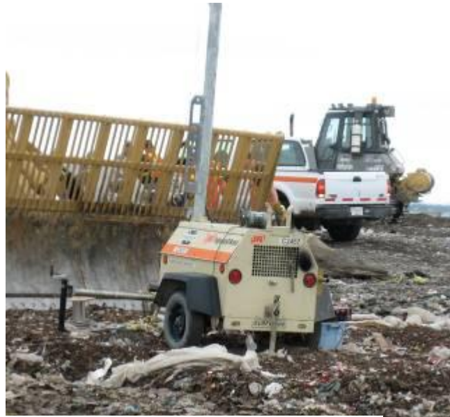
Fig 7: Portable lights in main dump are set up by Ops II workers.
