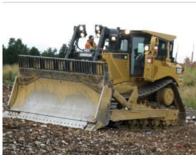
Fig 2: Ops II worker climbing out of the bulldozer at the demolition dump.
