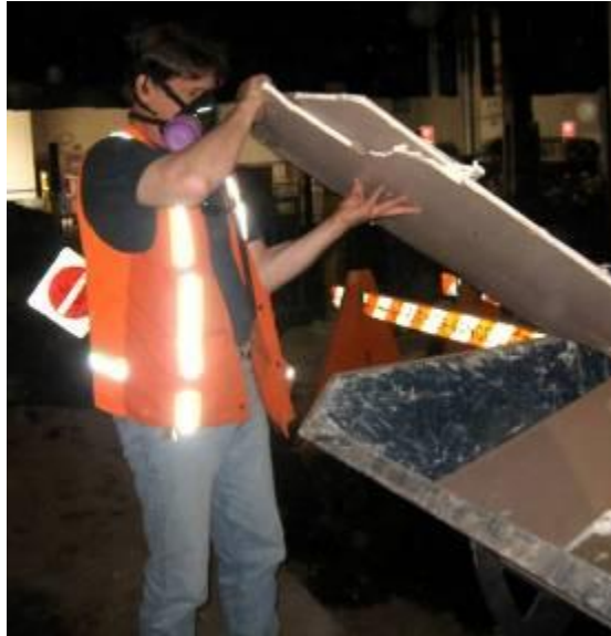
Fig. 9: Worker handling drywall set aside in a special bin.
