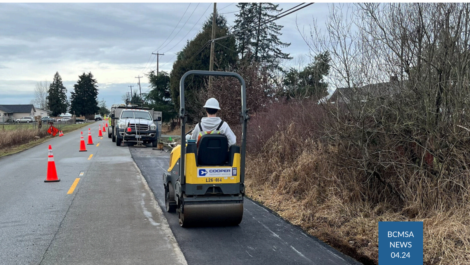
Image Below: Roads & Drainage Construction Crew, City of Surrey
